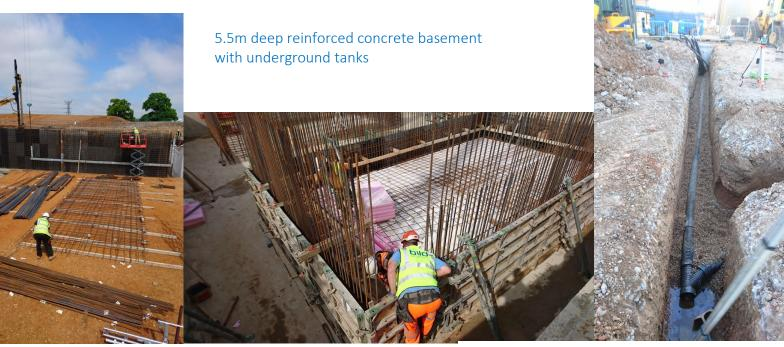
100m³ underground reinforced concrete leachate tank
